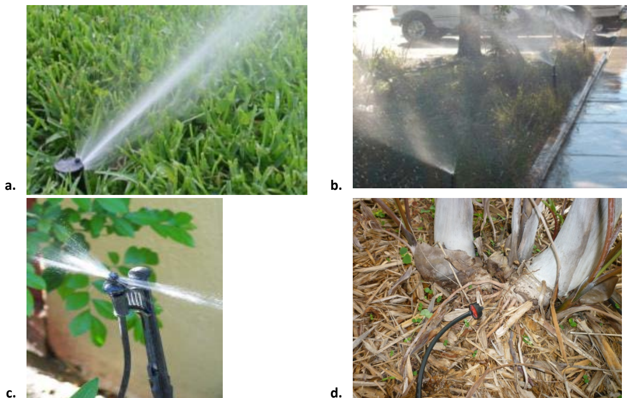
Figure 12. The three main categories of irrigation sprinklers: a) rotor, b) sprayhead emitter, and c and d) micro-irrigation emitters.
