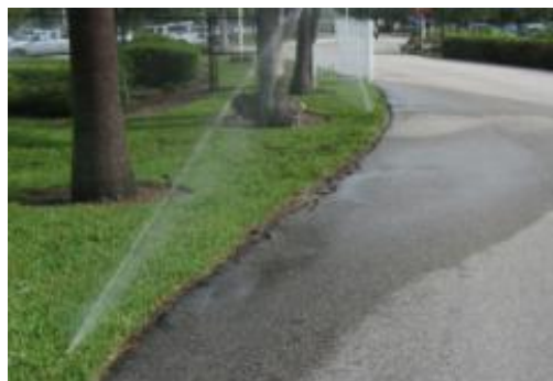
Figure 13. Sprinklers with a poor wetting pattern.
